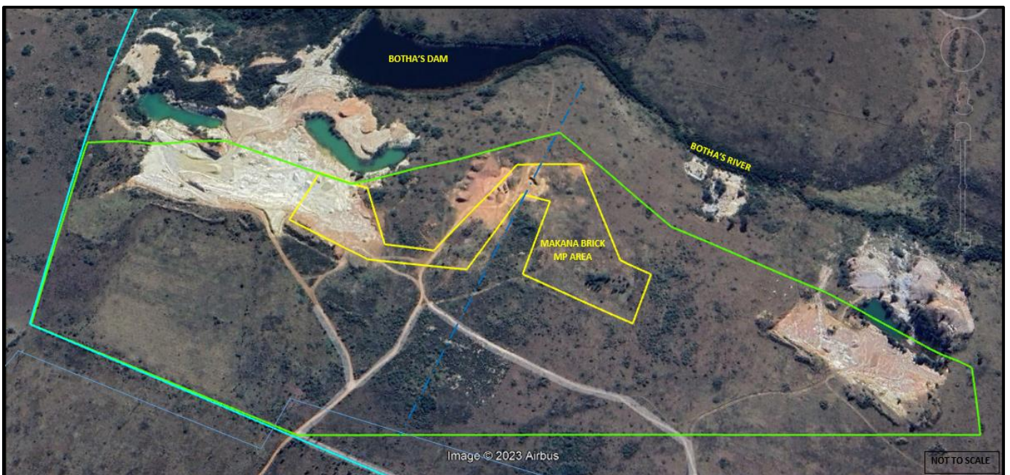
Figure 4: Satellite view of the Eskom power lines where the dotted blue line indicates the low voltage power line crossing the proposed mining area, and the solid blue line refers to the high voltage power line (image obtained from Google Earth).
